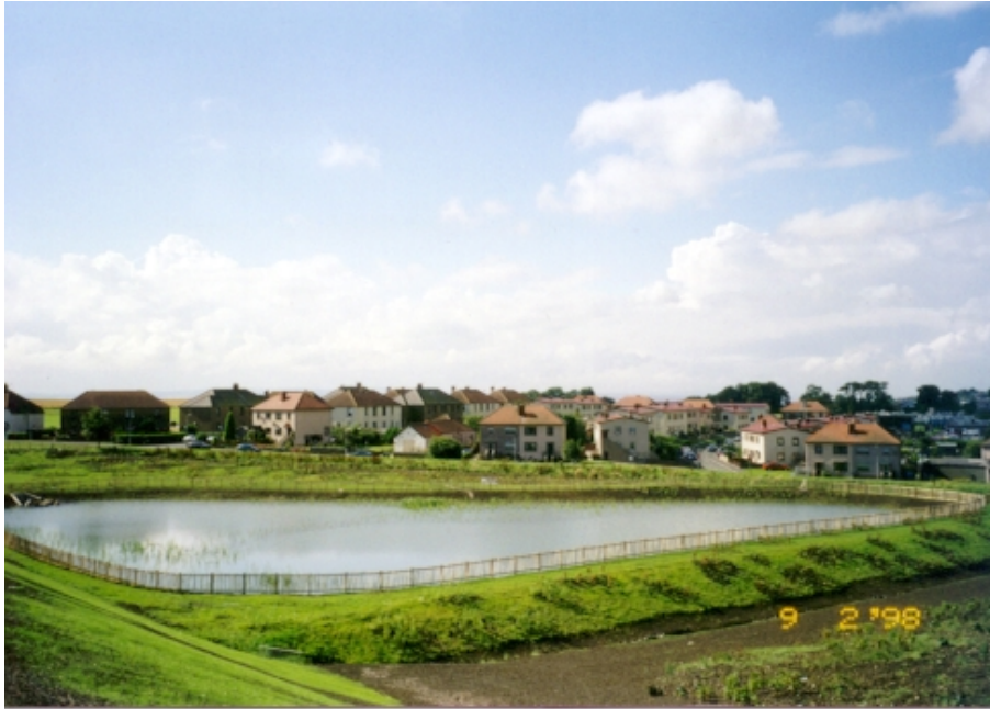
Figure 4.1 Wet stormwater pond near Edinburgh, Scotland. Inlet to the pond is on the left. The pond provides storage and treatment of urban and highway runoff.
