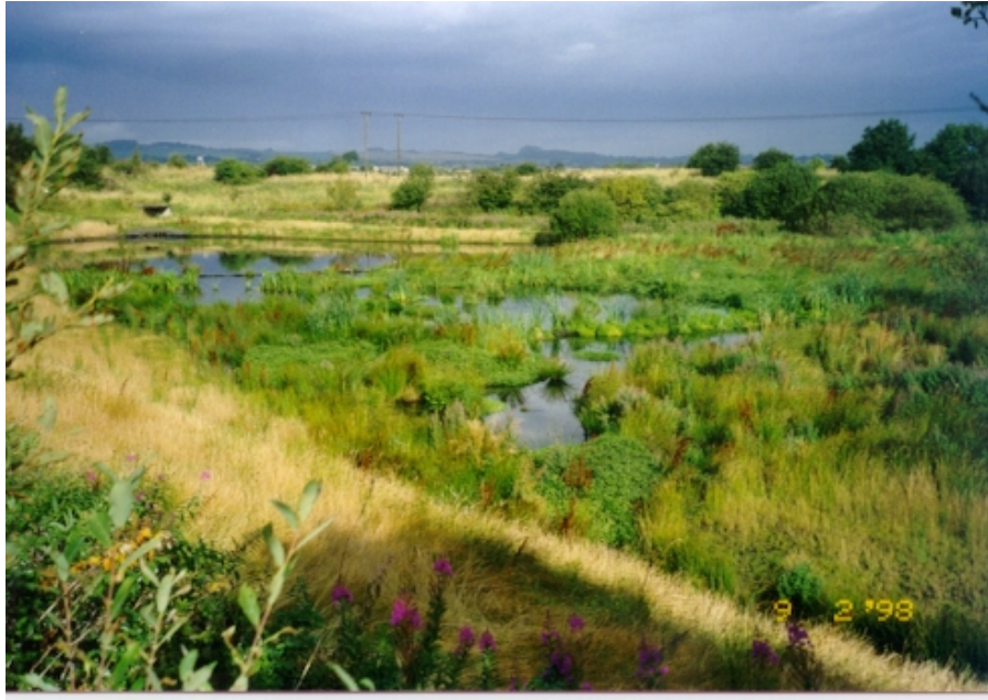
Figure 4.5 a Upstream view of a stormwater treatment wetland near Edinburgh, Scotland. The wetland consist of three pools in a series. The upstream pool is a shallow pond, the middle pool has standing water, and the third pool is made of reed basin.
