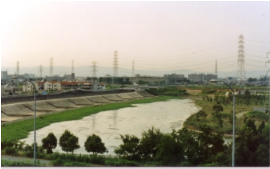
Figure 4.2 Off-line retention pond in Osaka, Japan. The river is behind the concrete spillway in the middle left side of the figure. The retention is activated when the flood level in the river exceeds the crest of the spillway. The water is pumped back from the storage after the flood event.
