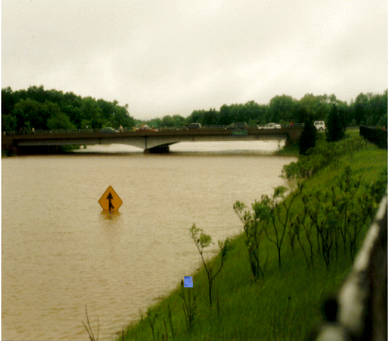
Figure 1.3. June 1997 flooding of Interstate 43 in northern Milwaukee metropolitan area. The event causing flooding was greater than 100 year storm. The capacity of an inverted siphon conveying a small suburban stream under the freeway was insufficient to handle the flow increased by urbanization.
