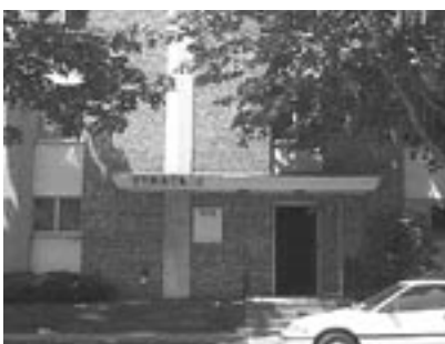
Strack II – 911 North 17th Street
